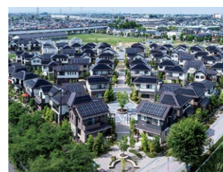
BRIDGE LIFE Platform 南栗橋
